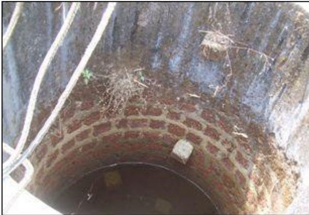
Photo 15: Ground water level in the open dug well at the toe part of the Sasanwad slide.
