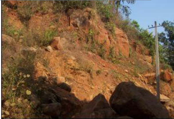
Photo 1: A view of Sasanwad slide no-1.
