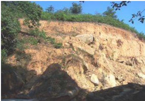
Photo 3: A view of Sasanwad slide no-3.
