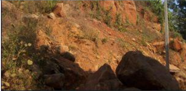
Photo 13: Prominent set of joint in Gneiss outcrop on the right flank of the Sasanwad slide no-2.
