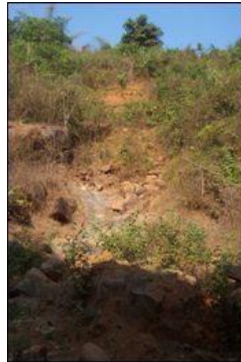
Photo 2: A view of Sasanwad slide no-2.
