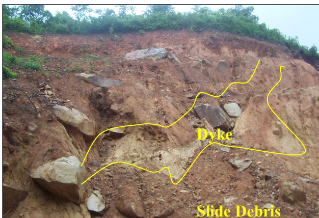
Photo 5: view of dyke exposure in Sasanwad slide no-3.
